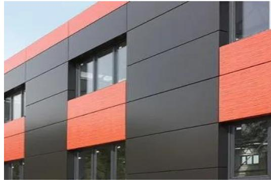
The growth of ACP product use over the last 10 years, particularly in high rise applications, has been attributed to its light weight and aesthetic qualities. ACPs do not generally add to the structural integrity of a building but may contribute to the energy efficiency and weather proofing of an external wall.
